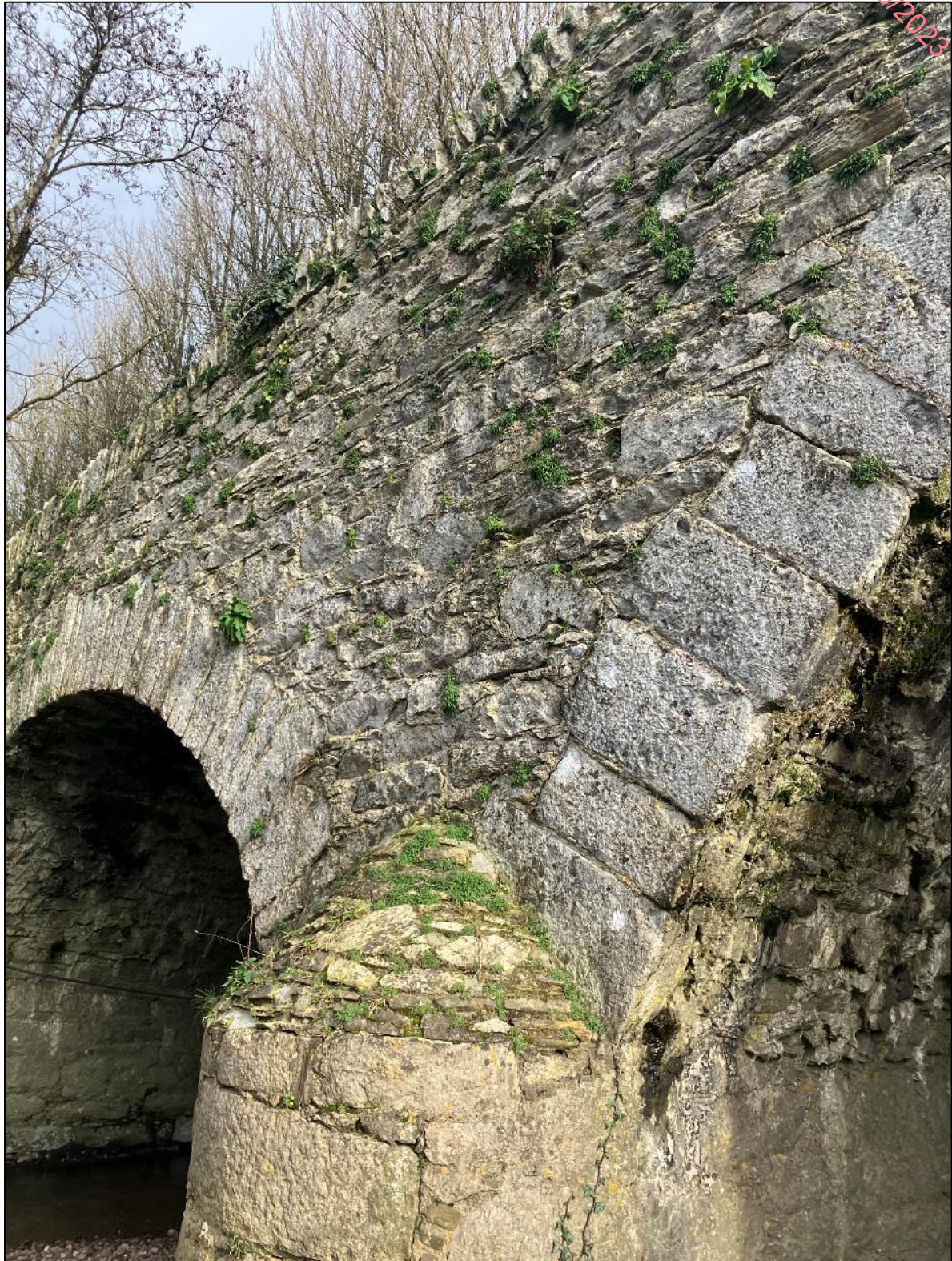
Image 3: Pier/ Cutwater Between Arch 2 & 3
