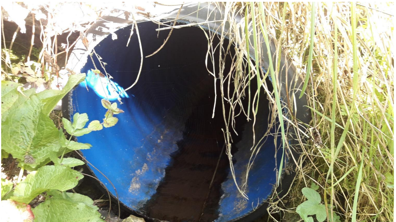
Image 16: Twin wall drainage pipe installed in a masonry box culvert.
