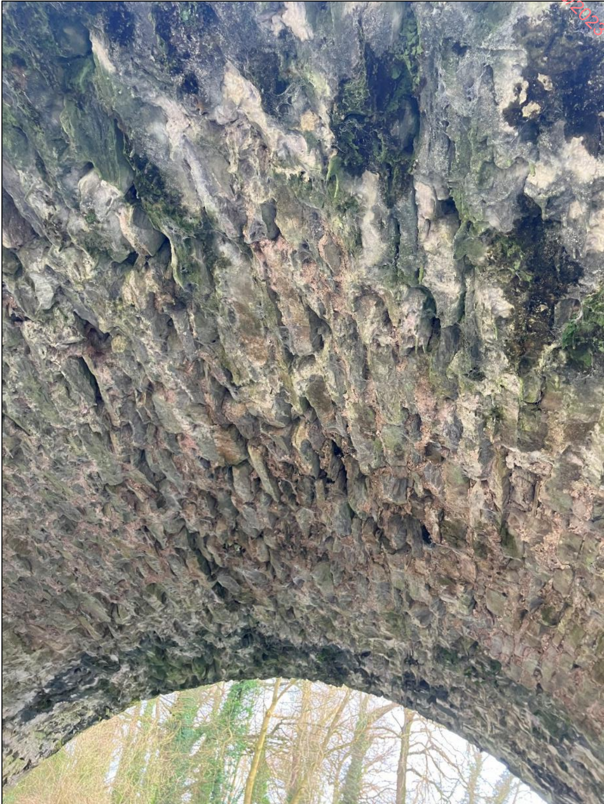
Image 5: Cavities at apex of barrel of Arch 2.
