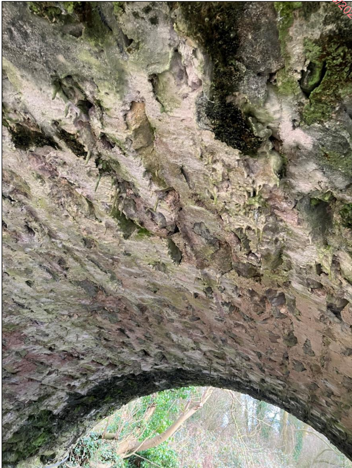
Image 7: Cavities at apex of barrel of Arch 3.
