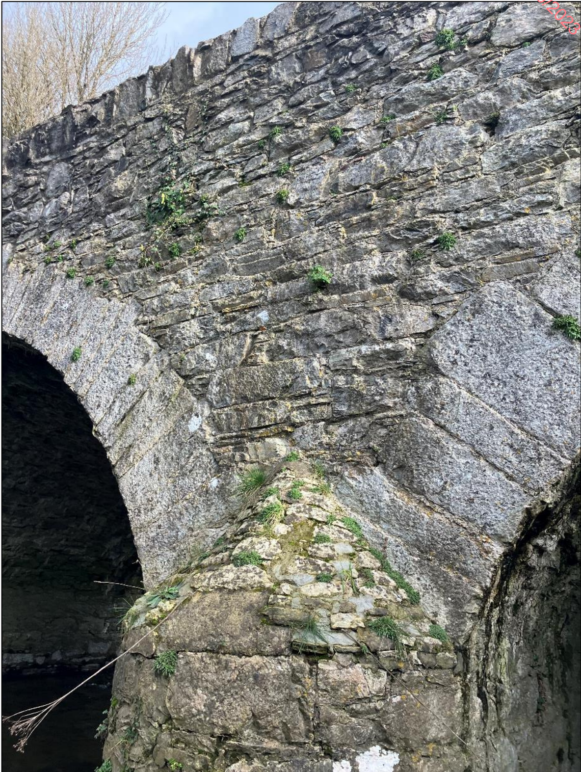
Image 2: Pier/ Cutwater Between Arch 1 & 2
