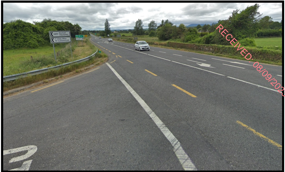
Figure 2.8 - Existing N72/R671 Junction
