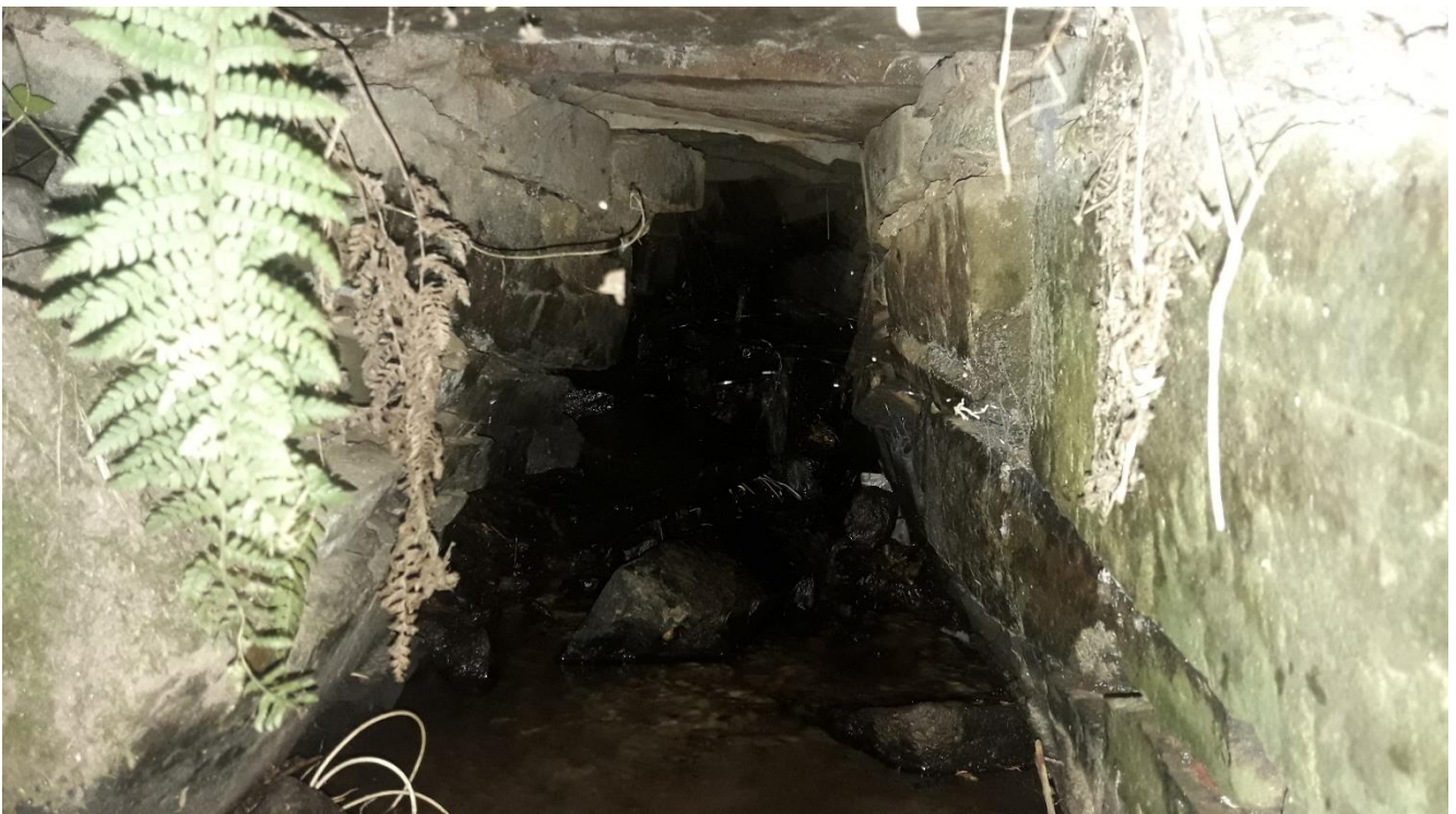
Image 11: Masonry Box Culvert.
